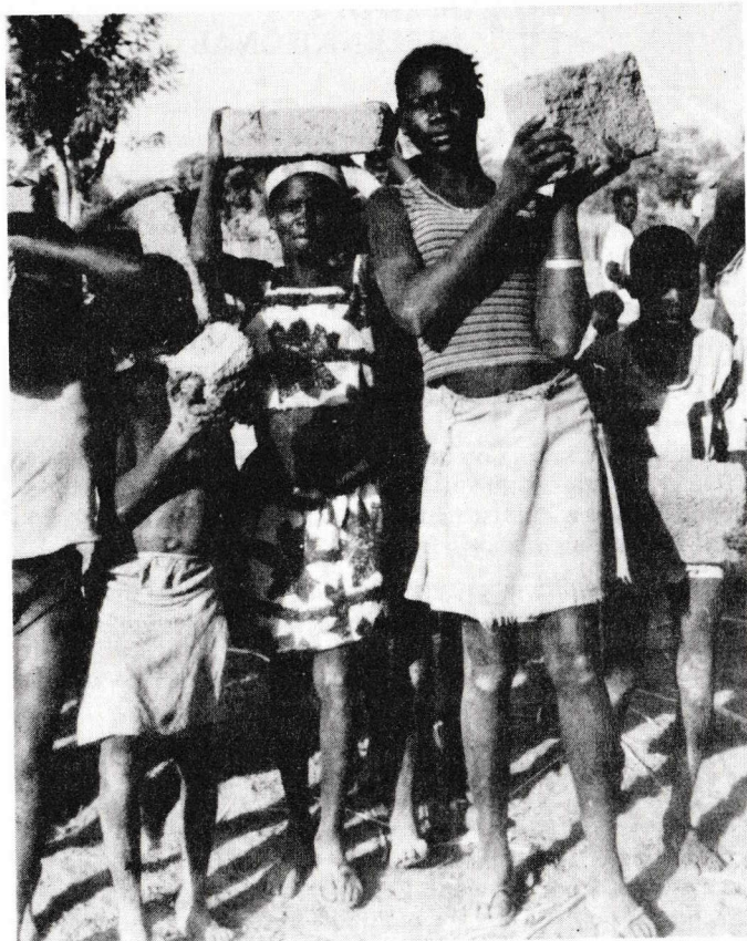
Carrying bricks for building the Grain Silo, Upper Volta.
